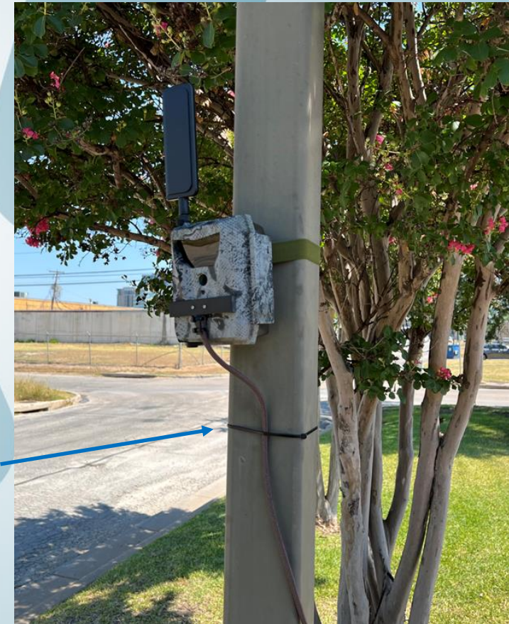
Camera and Eyepatch Deployment with Strain Relief
