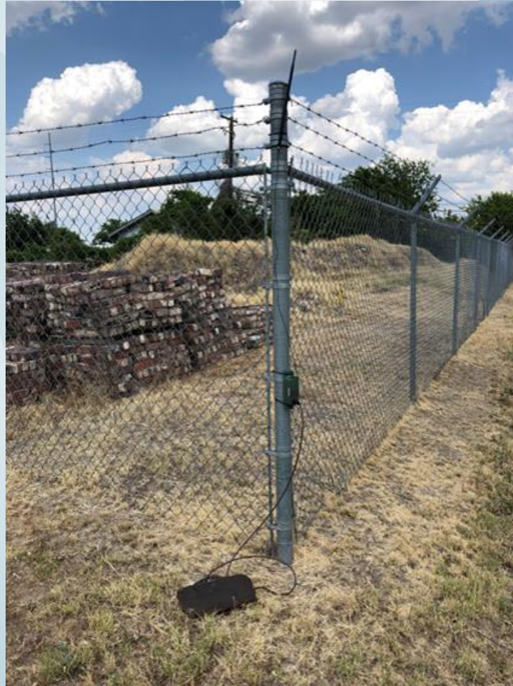
Fence Post Installation
