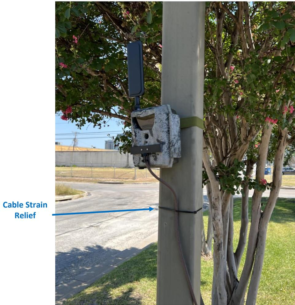
Figure 14: Eyepatch Module Strain Relief
