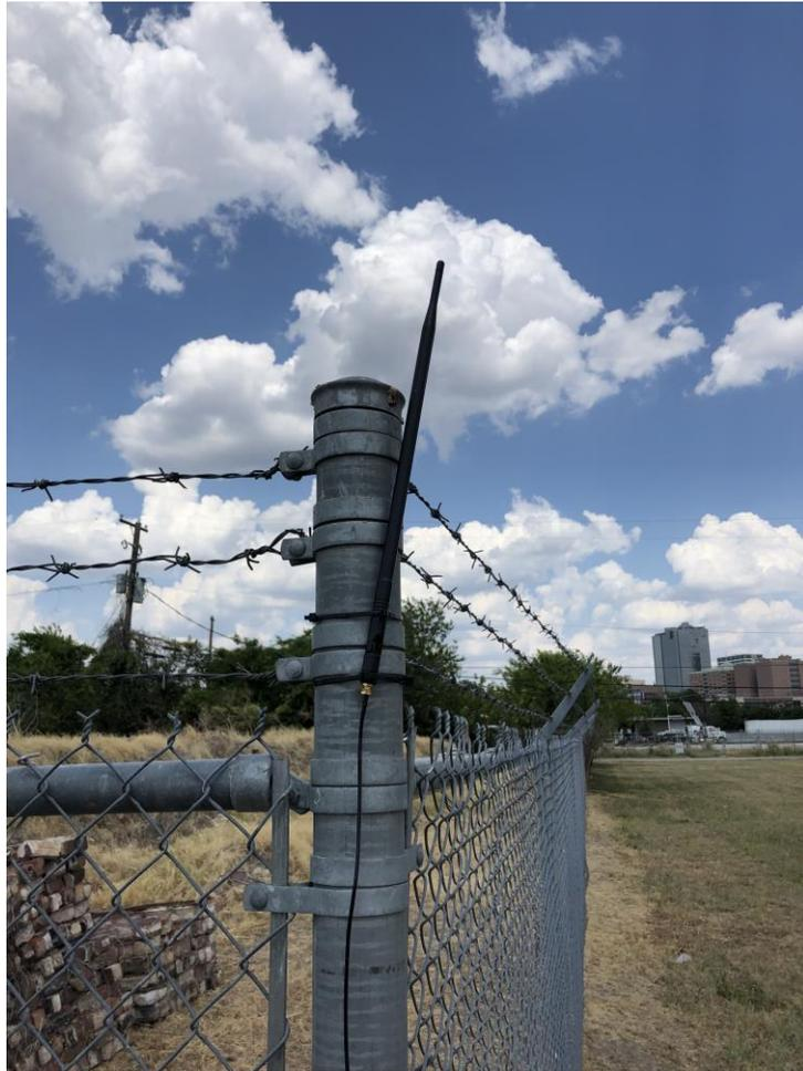
Figure 49: Antenna Mounted to a chain link Fence
